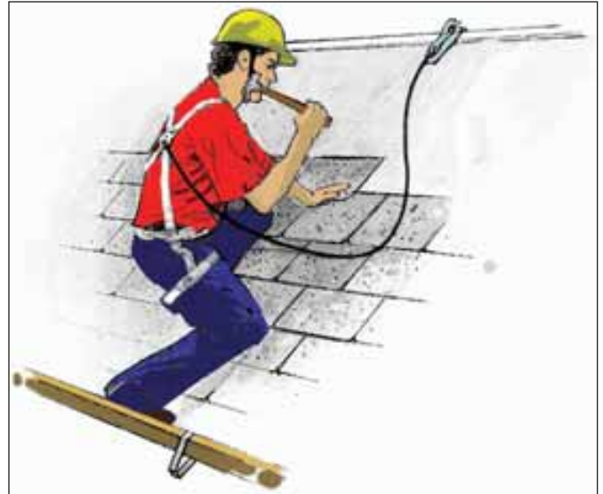
An example of a worker using both fall restraint equipment and a toe-hold.
