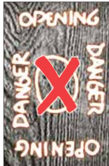
Examples of markings on a plywood cover.
